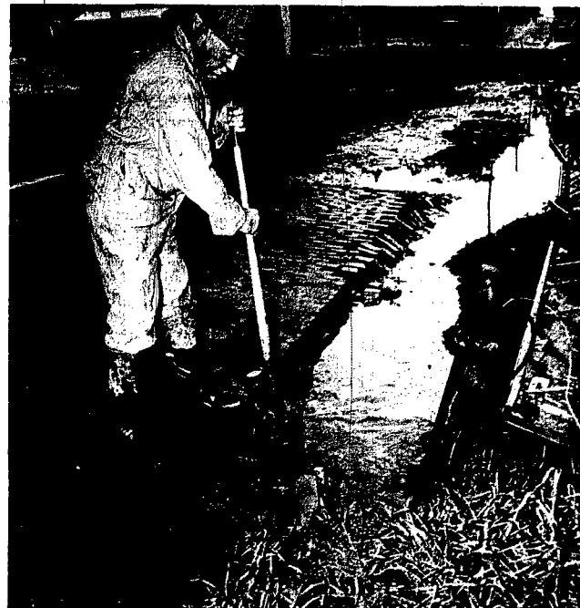
FRED HAAS, Pierce, appears to be rowing a freight barge upstream at the intersection of 7th and Main. Actually, he was one of a crew attempting to dissipate rain water Friday morning. Heavy rains during the week halted the street improvement project, delaying its completion.
